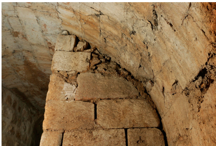
Figure 22. Photo of the first buttress against the south wall of the original chamber.
