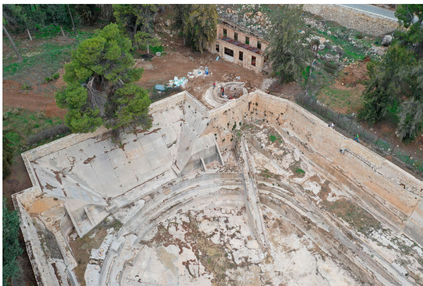
Figure 7. Photo of the northwest corner of the Lower Pool showing examples of the interior terraces of the pool. The large portion of the South Wall that is part of the British Mandate renovation. Note the sloping channel into the pool at centre.
