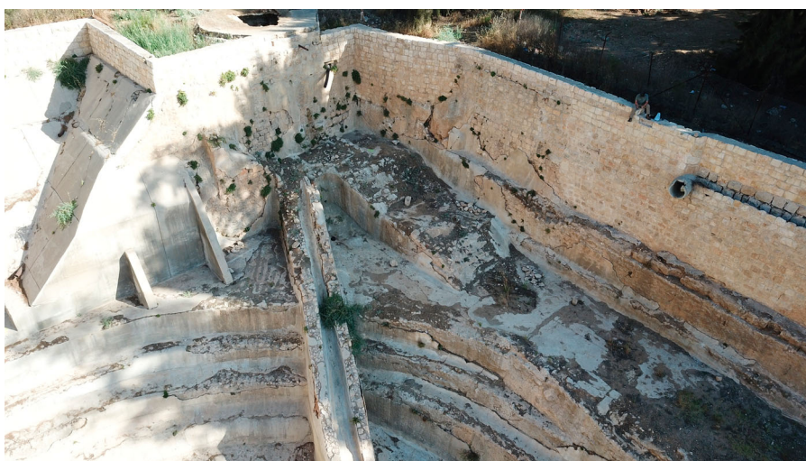
Figure 11. Photo of northwestern corner of the Lower Pool. Note the traces of two basins (filled with earth) at the top of the sloping channel and the wide staircase.
