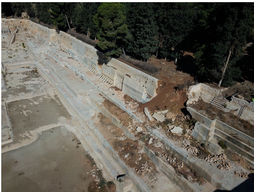
Figure 6. Photo of the collapsed portion of the North Wall of the Lower Pool.
